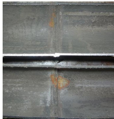
Figure 5: Girth Weld Area (Internal)
